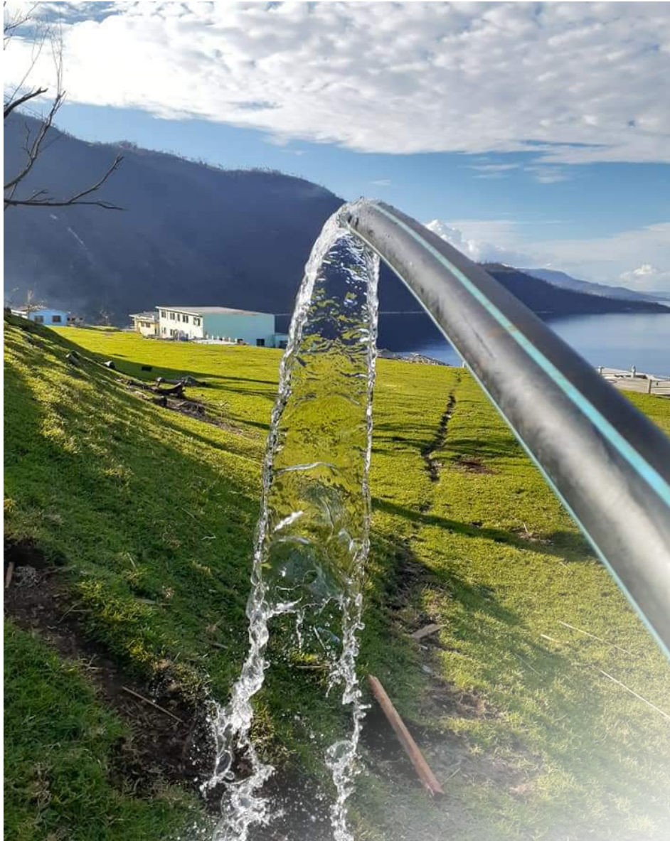
Source: Vanuatu Department of Water Resources. Water being reconnected in Pentecost.
