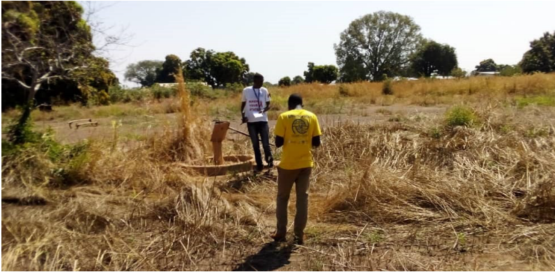
Abu-shaka non functional borehole © IOM 2019
