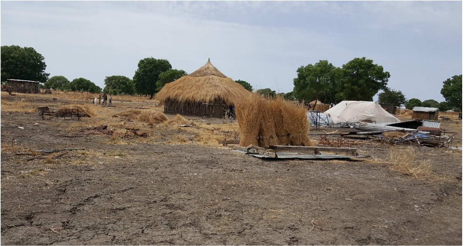
Returnees rehabilitating shelters in Makuach (Bor South County) ©IOM 2019
