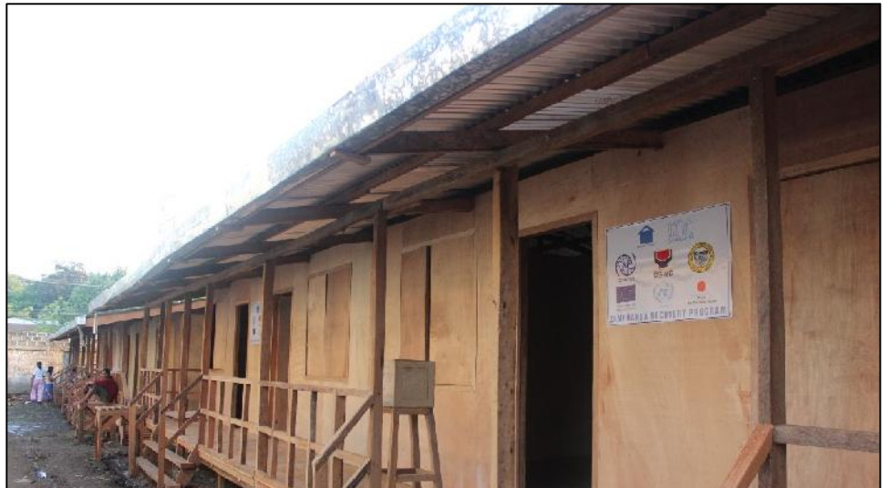
The seven units of bunkhouses with 12 rooms in each bunkhouse PTSI Transitory Site is ready to shelter IDP families.
