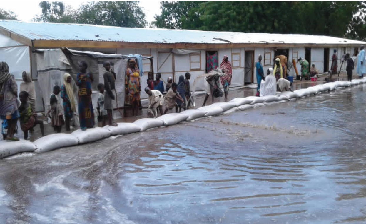
Above are Pictures taken at the site showing damaged shelters and flooded areas.
